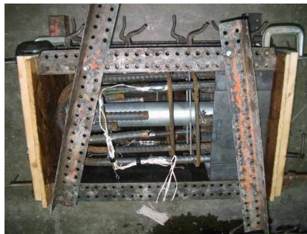
Figure 39. Photograph of Column 2 reinforcement in forms.
