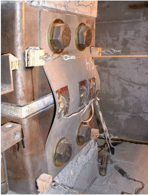
a.) West fuse plate buckling
