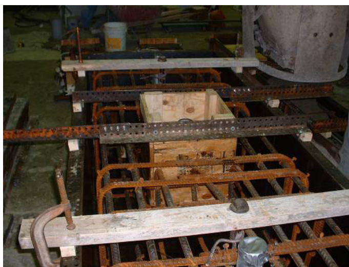
Figure 50. Photograph of Column 4 foundation reinforcement in forms.
