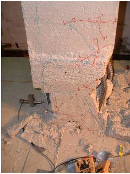
a.) South view of damage
