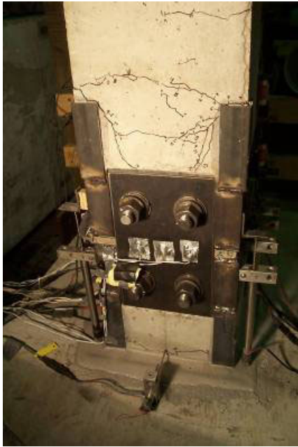
a.) East face crack progression
