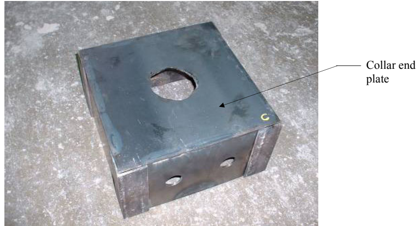
Figure 41. Photograph of Column 3 collar and end plate.
