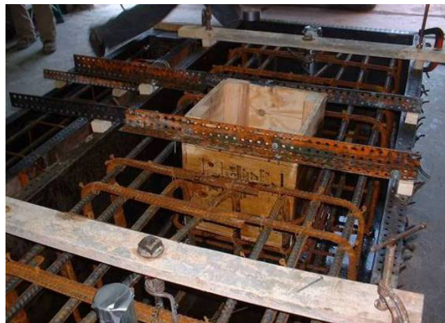
Figure 49. Photograph of Column 3 foundation reinforcement in forms.
