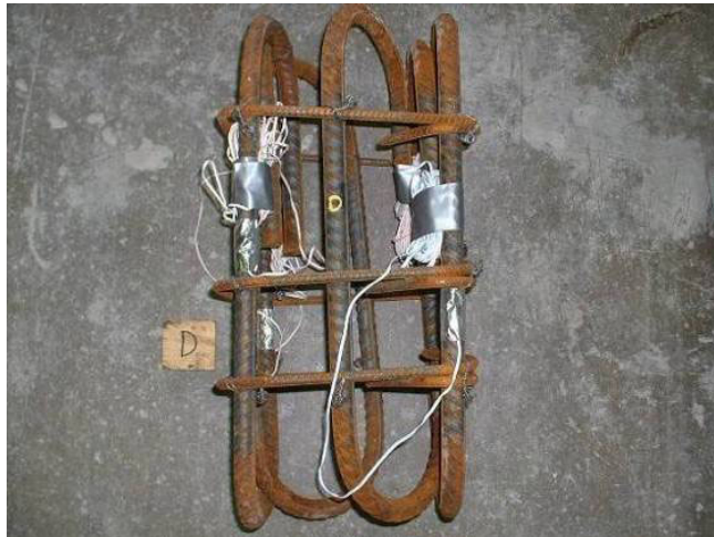
Figure 42. Photograph of Column 3, 2 ft. segment reinforcement.
