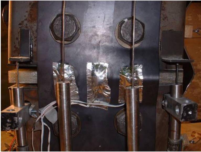
a.) North fuse plate differential buckling
