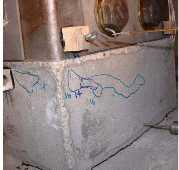
b.) Northwest corner compression damage
