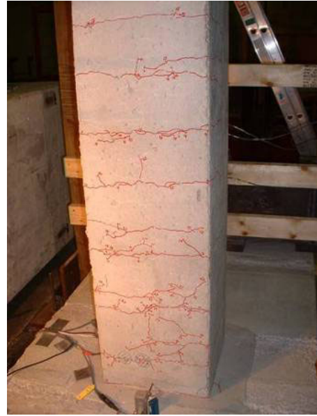
b.) East face crack progression
