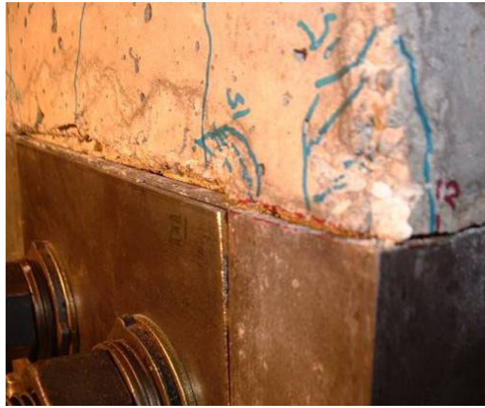
b.) Northeast corner collar/column interface
