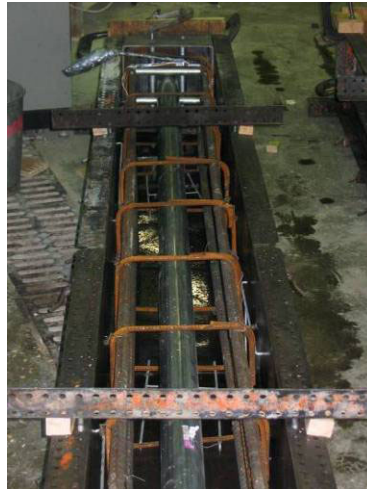
Figure 59. Photograph of Column 6 in forms.
