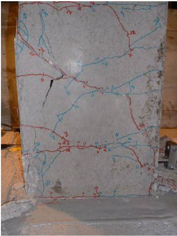
c.) North face cracking/spalling
