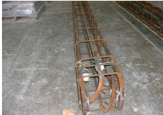
Figure 48. Photograph of Column 4, 12 ft. segment reinforcement.
