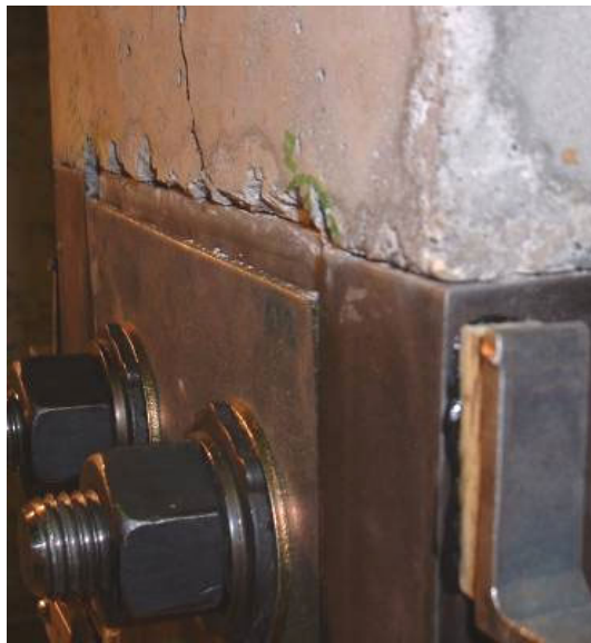
a.) Northeast corner interface opening
