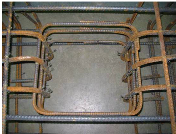
Figure 25. Photograph of center socket reinforcement.
