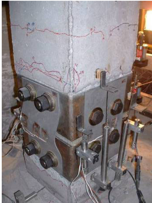
Figure 155. Photograph of Column 6 – Cycle 26b, column damage.
