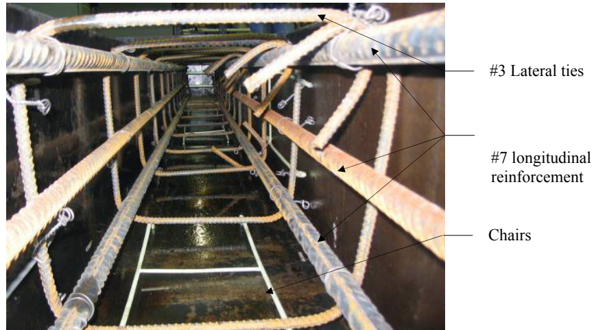
Figure 31. Photograph of chairs and reinforcement in Column 1.
