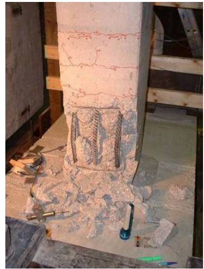
b.) East face reinforcement exposed
