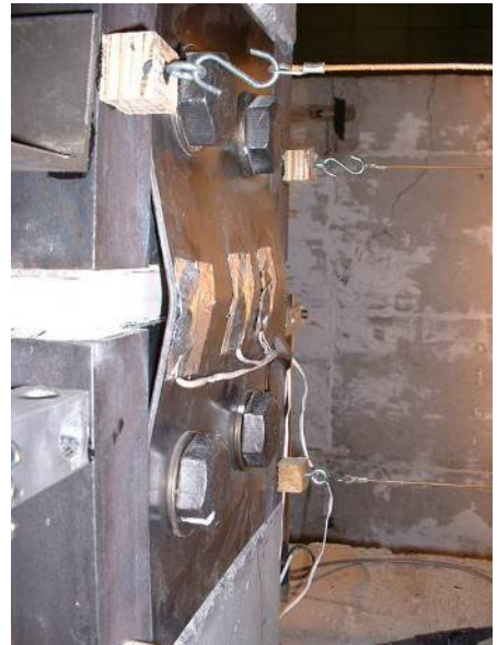
d.) Buckling of replaced west plate
