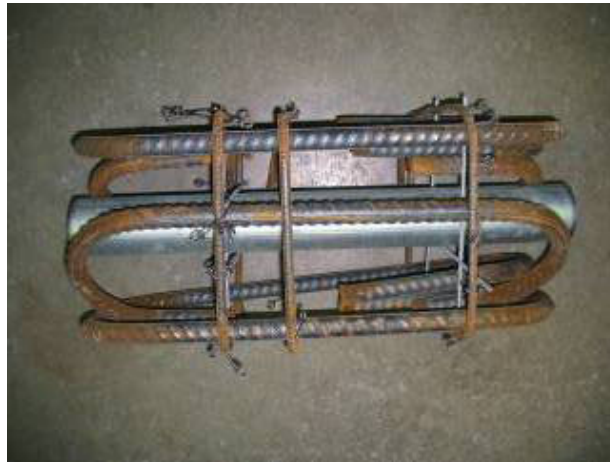
Figure 38. Photograph of reinforcement of Column 2 (2 ft. column segment).
