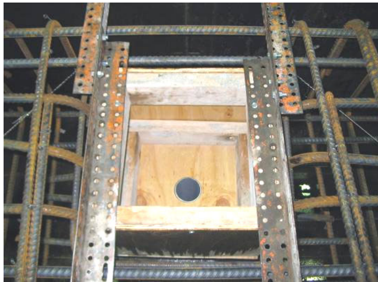
Figure 29. Photograph of boxout in forms.
