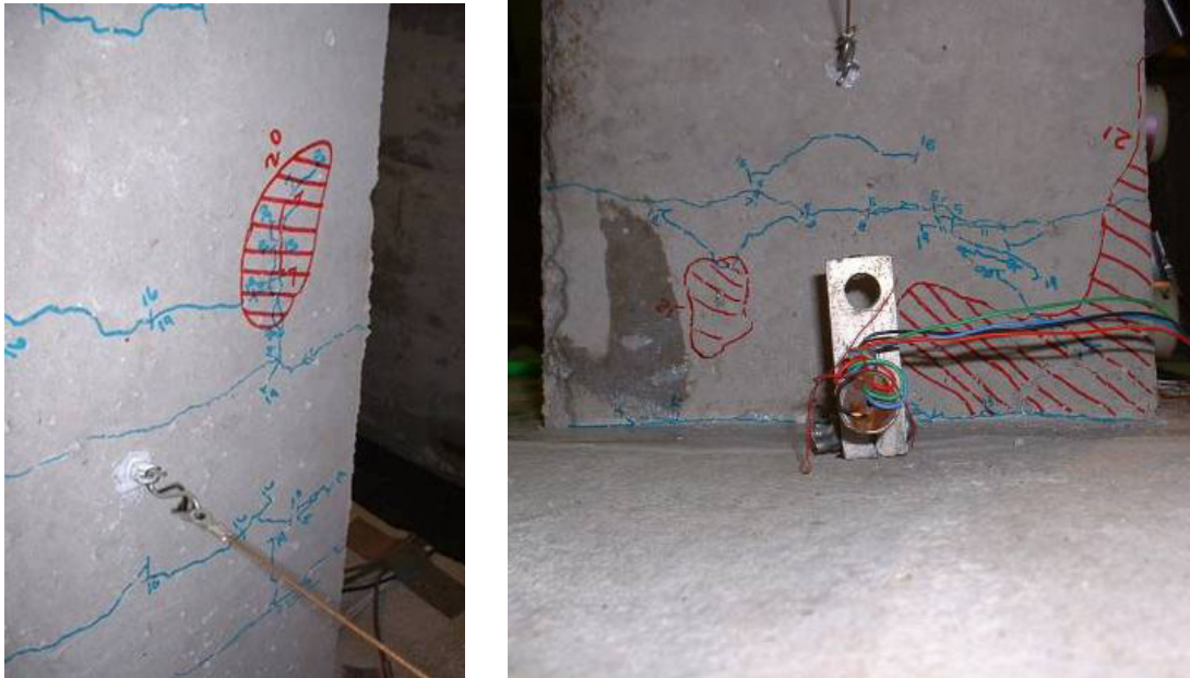
a.) West face initial compression damage b.) Localization of compression damage on southwest corner
