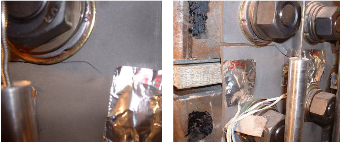
a.) Initial fracture of south fuse plate at -5.22 in. displacement b.) Fuse plate crack at -9.0 in. displacement
