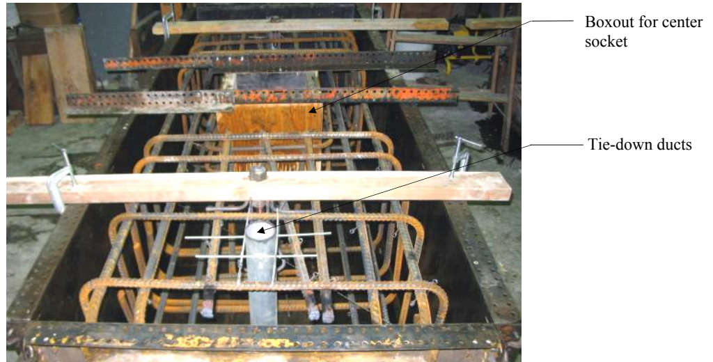
Figure 28. Photograph of foundation reinforcement and tie-down ducts in forms.
