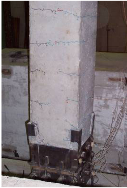
a.) Northwest corner damage
