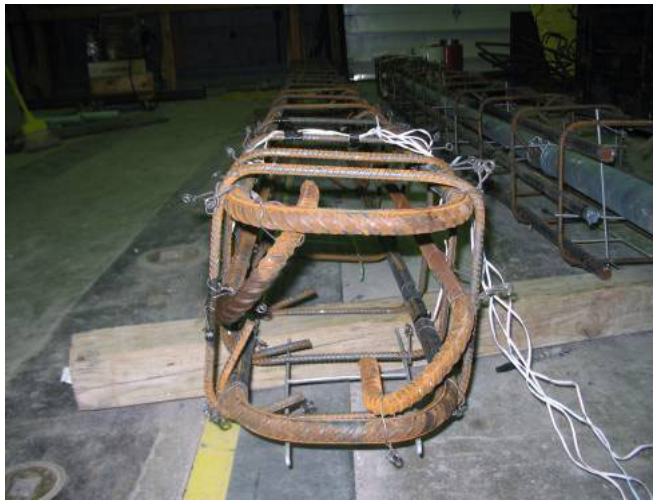
Figure 15. Base end of control column reinforcement cage.
