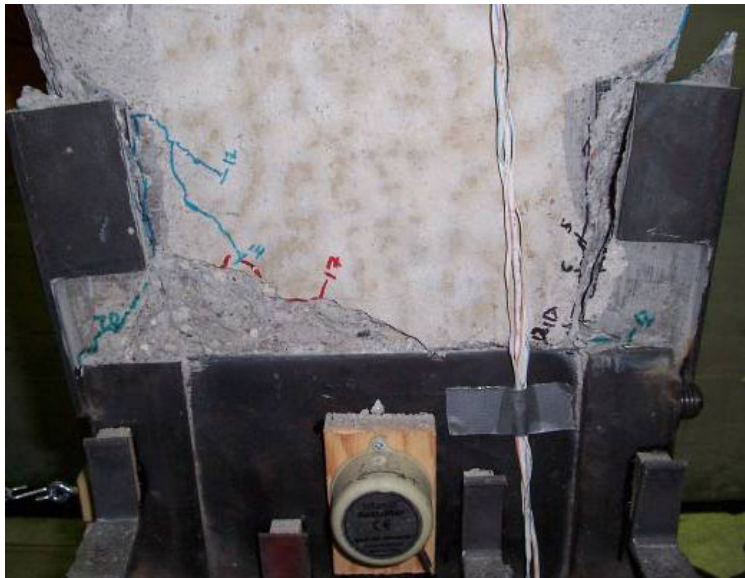
a.) South side view of retrofit angle failure
